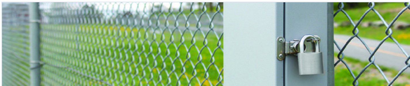
VCS-600 weatherproof processor on the fence line
